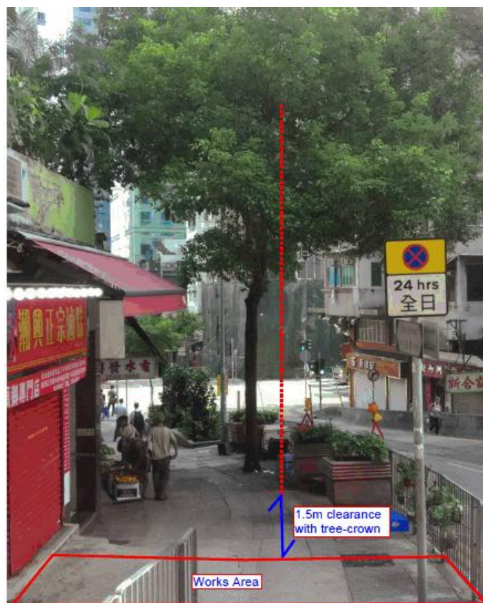
Photo 1: Vertical clearance between tree-crown and works area
